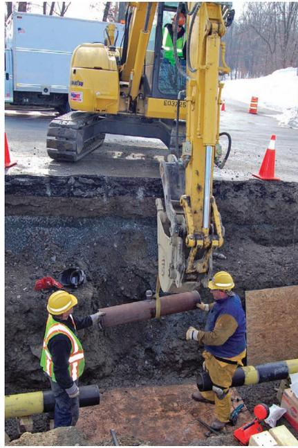
**Gas crews repair a natural gas line damaged by a non-utility contractor. The damage affected service to two towns.**
